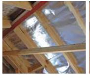
FOIL INSULATION Reflects the suns heat and creates a thermal barrier to keep into the roof space the home cool. Fire retardant foil insulation is manufactured from highly burnished aluminium foil bonded with flame retardant adhesive to a woven polymeric mesh.
