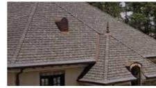
Bitumen, or asphalt, shingles are made from paper and fibreglass, coated with bitumen and asphalt, and ceramic granules. Expensive to install as they need a plywood deck & each tile needs fixing individually. Susceptible to fire and heavy rainfall causes permanent damage. UV damage means frequent replacement.
