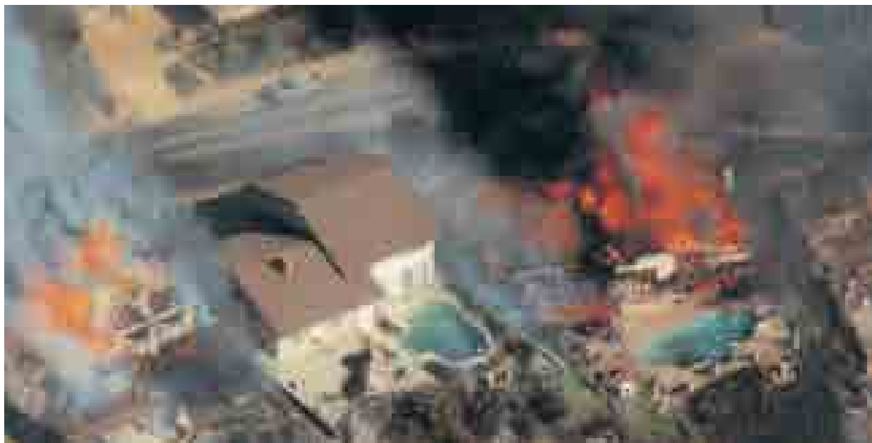
ABOVE: DURING A MAJOR CALIFORNIAN BUSHFIRE, THIS SUBURB WAS IN FLAMES, PASSING FROM ROOF TO ROOF BY FLYING EMBERS. MOST HOMES WITH STEEL TILE ROOFS ESCAPED.
