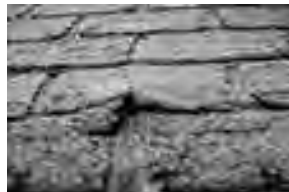
ASPHALT SHINGLES DAMAGE
