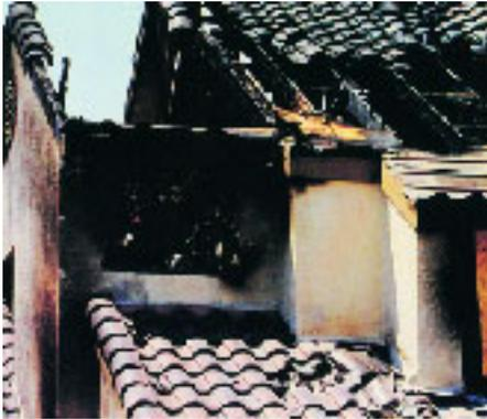
■ Orange, California. This home was completely destroyed by an interior fire. As the fire burned the heavy tile roof began to collapse. With concrete tiles now becoming a danger, the Fire Department was unable to fight the fire from within the house.
