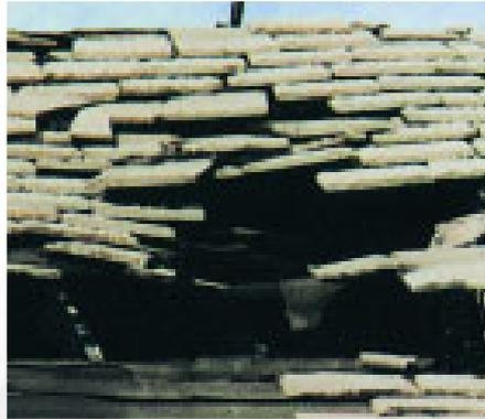
■ This roof at 30kg/m<sup>2</sup> is over four times heavier than tiles made by AHI Roofing. There is an added danger of the fire-weakened rafters collapsing under the weight of the roof, both during and after the fire.
