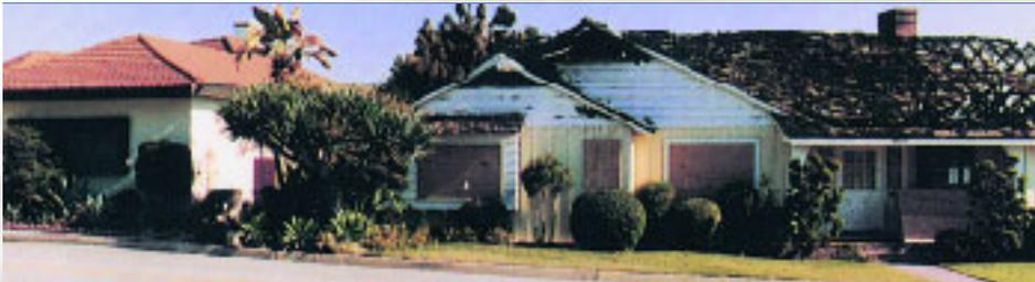
■ The home on the left was re-roofed with tiles from AHI roofing. More than 50 surrounding houses burned. Although the fascia boards blistered and charred, and windows cracked in the severe heat, the house with the roof from AHI Roofing did not burn.
