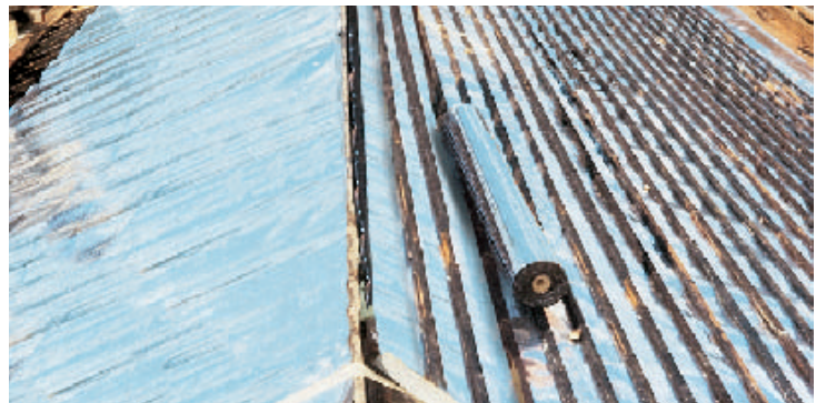
AHI foil installed under battens.
