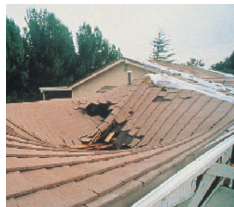
These cement shakes slipped causing sub-structural damage
