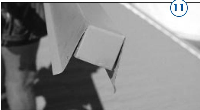
Then continue up the roof, bending and tacking trims as you go. On completion, check for straightness, and nail fast.
