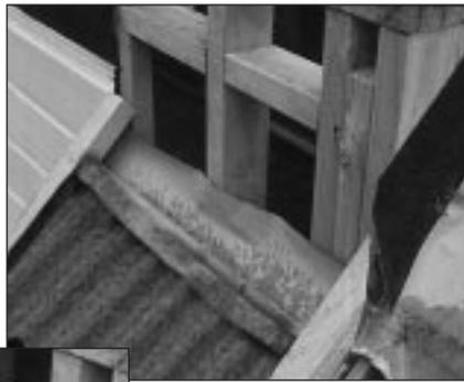
Cut and bend last tile to fit flush with the wall. A support batten is recommended at the foot of the wall.
