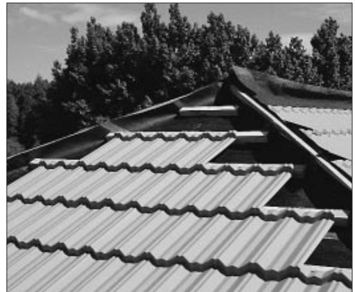
As each length of underlay is laid, replace the battens on the top of the building paper against the marking nails.
